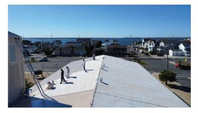
This is a photo of workers resealing the roof on Saint Catharine of Siena Church in Seaside Park last week. The men power-washed the roof before resealing the entire roof, which will extend the life of the roof for about 15-20 years. This project in now complete and paid for in-full through your generosity in the second collections for Parish Building Repairs.
